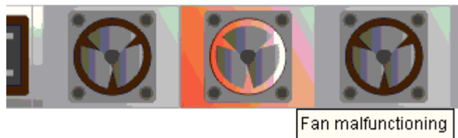
Figure 13-12: Cooling FAN Module malfunctioning message.
